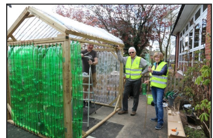
Feeding bottles onto canes and fixing to the frame
